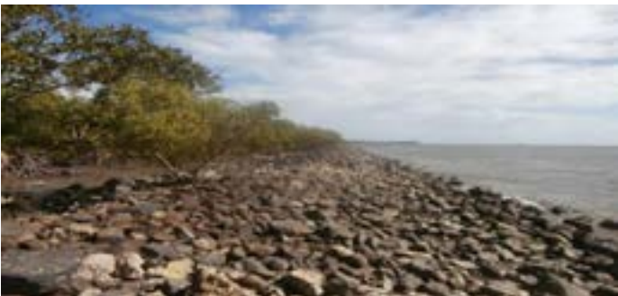
Figure 11. "Hampil" or artificial rock barriers established by the fisher folks and other people in the community to protect the growing mangrove trees in Brgy. Suclaran, San Lorenzo.
