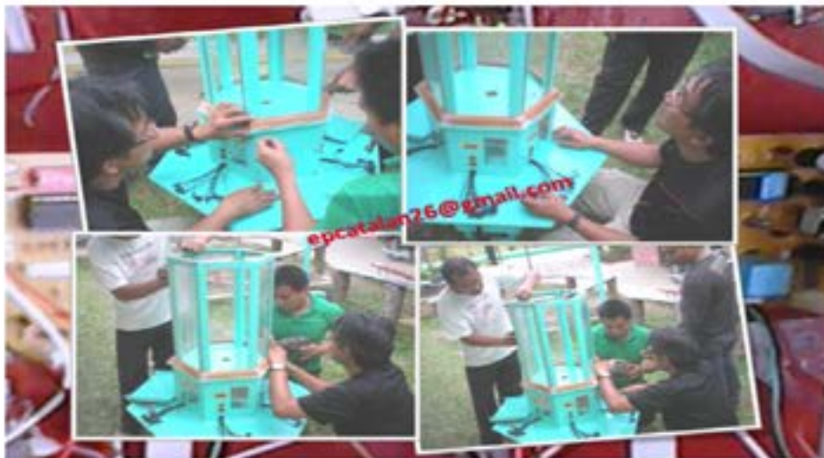
Figure 9. Assembling the charger structural frame of the charging station as shown in the picture.
