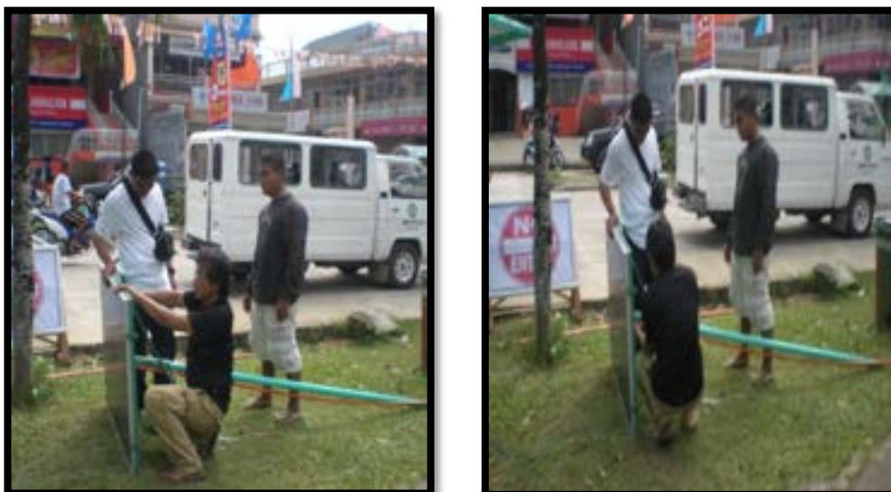
Figure 14. Assembling the solar (PV) panel as shown in the picture.
