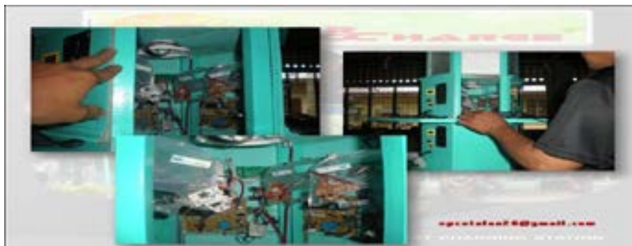
Figure 10. Completing the installation of the internal circuitry of the charging station.
