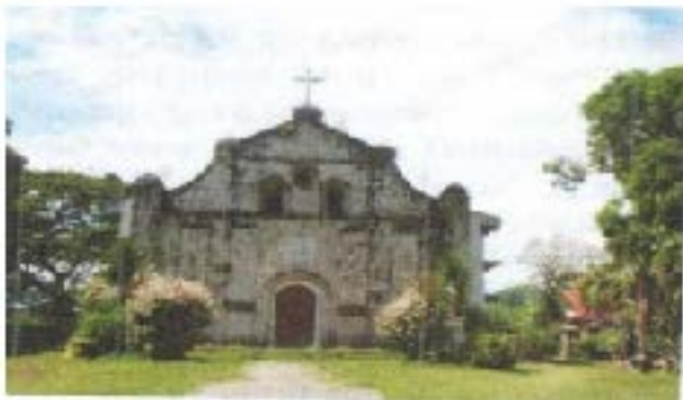
The Navalas Church built during the Spanish period.
