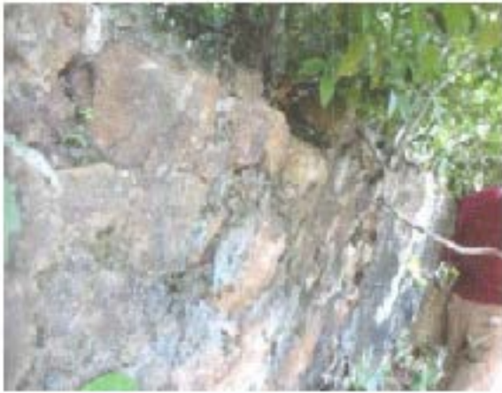
The close-up view of the parapet showing the materials used by the American soldiers to build it.
