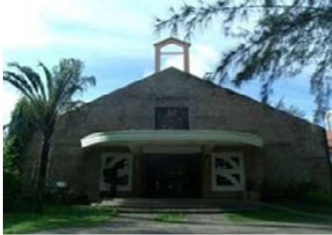
Fig. 12. The Trappist Monastery Church in Guimaras Island.
