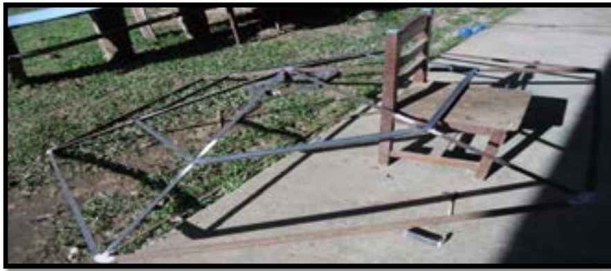
Figure 12. The top dome steel framing as shown in the picture.
