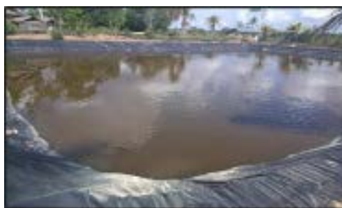
Photo: GST Gamo Fig. 1. SFR with HDPE Lining at Brgy. Nazaret, Buenavista
